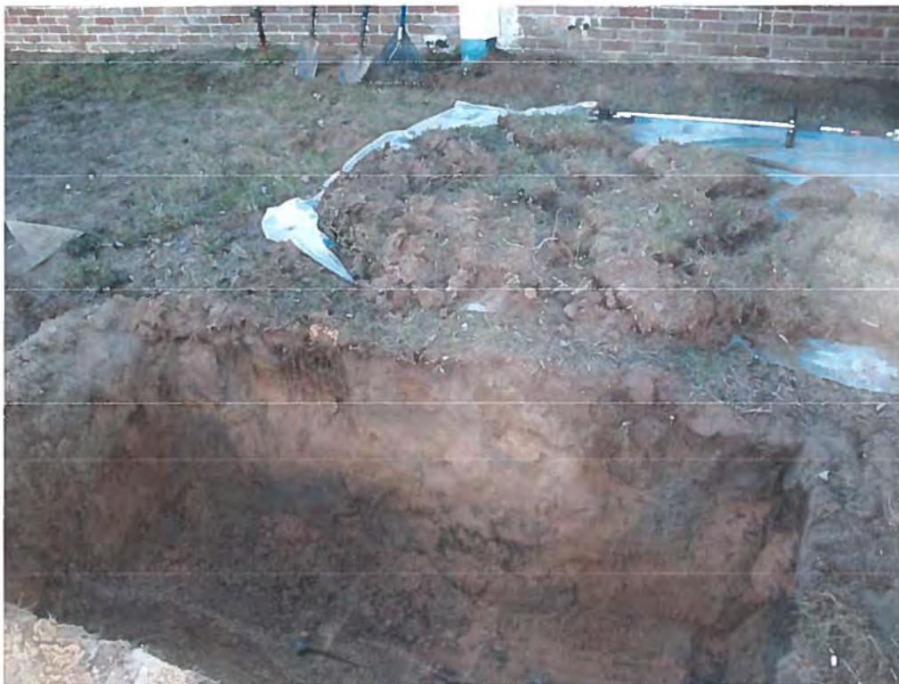
Picture 2: UST 881Cobia excavation in progress.
